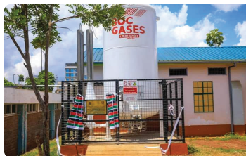
Liquid oxygen tank installation at kiambu level V hospital
